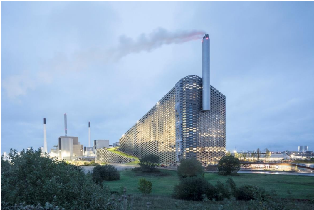
Figure 2.8. CopenHill Energy Plant and Urban Recreation Center / BIG, Copenhagen, 2019, photo by Laurian Ghinitoiu 104
