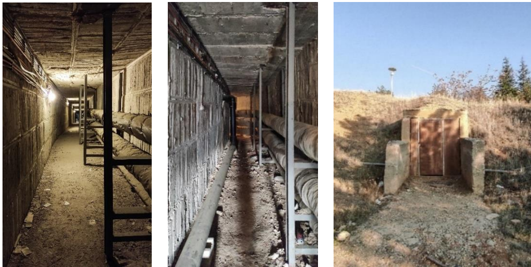
Figure 3.6. Photos from the gallery inspection, taken by the author
